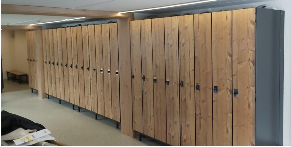
Further recently equipped locker rooms:
